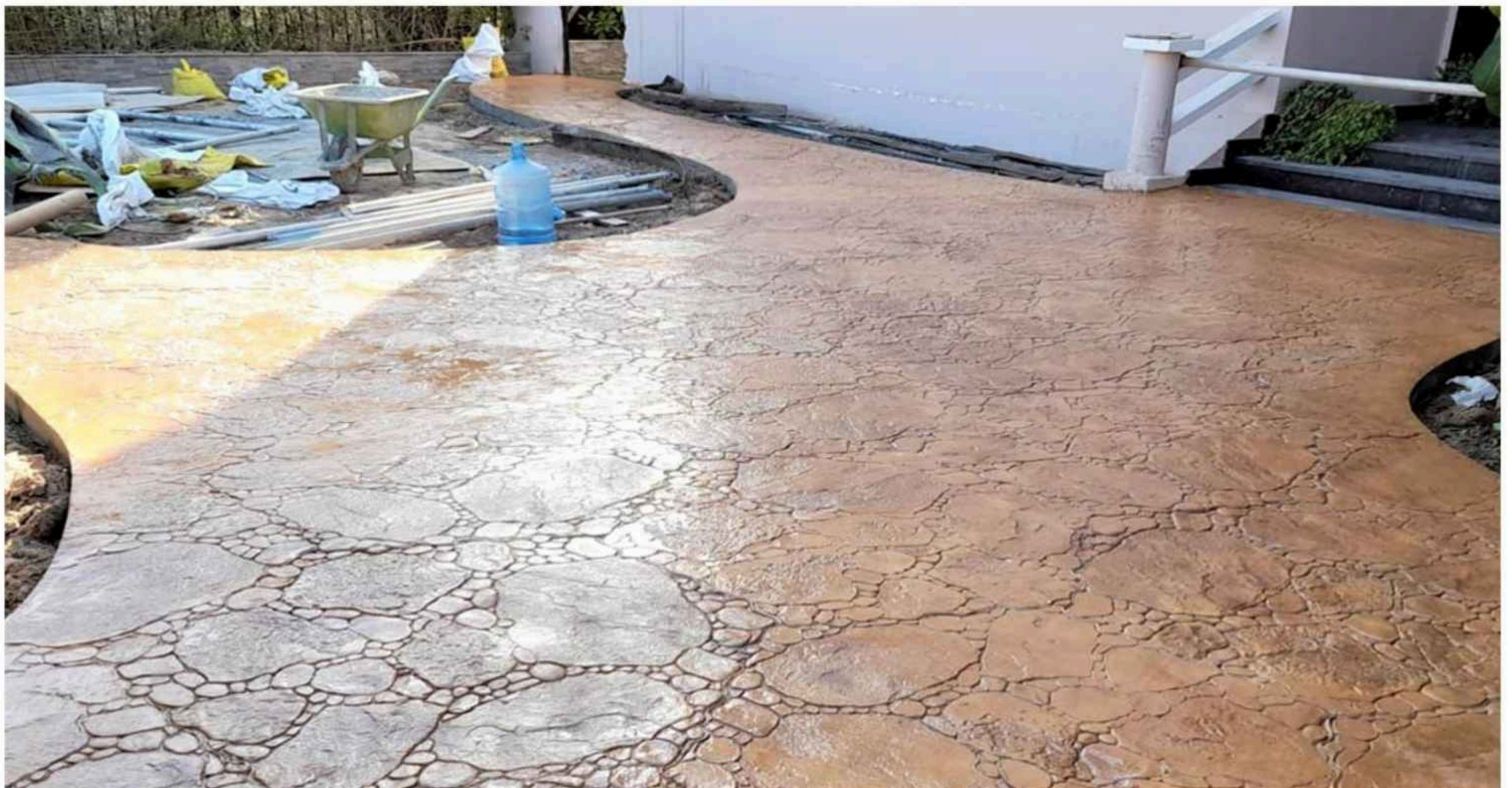
Stamped concrete work in The Villa, Dubai
