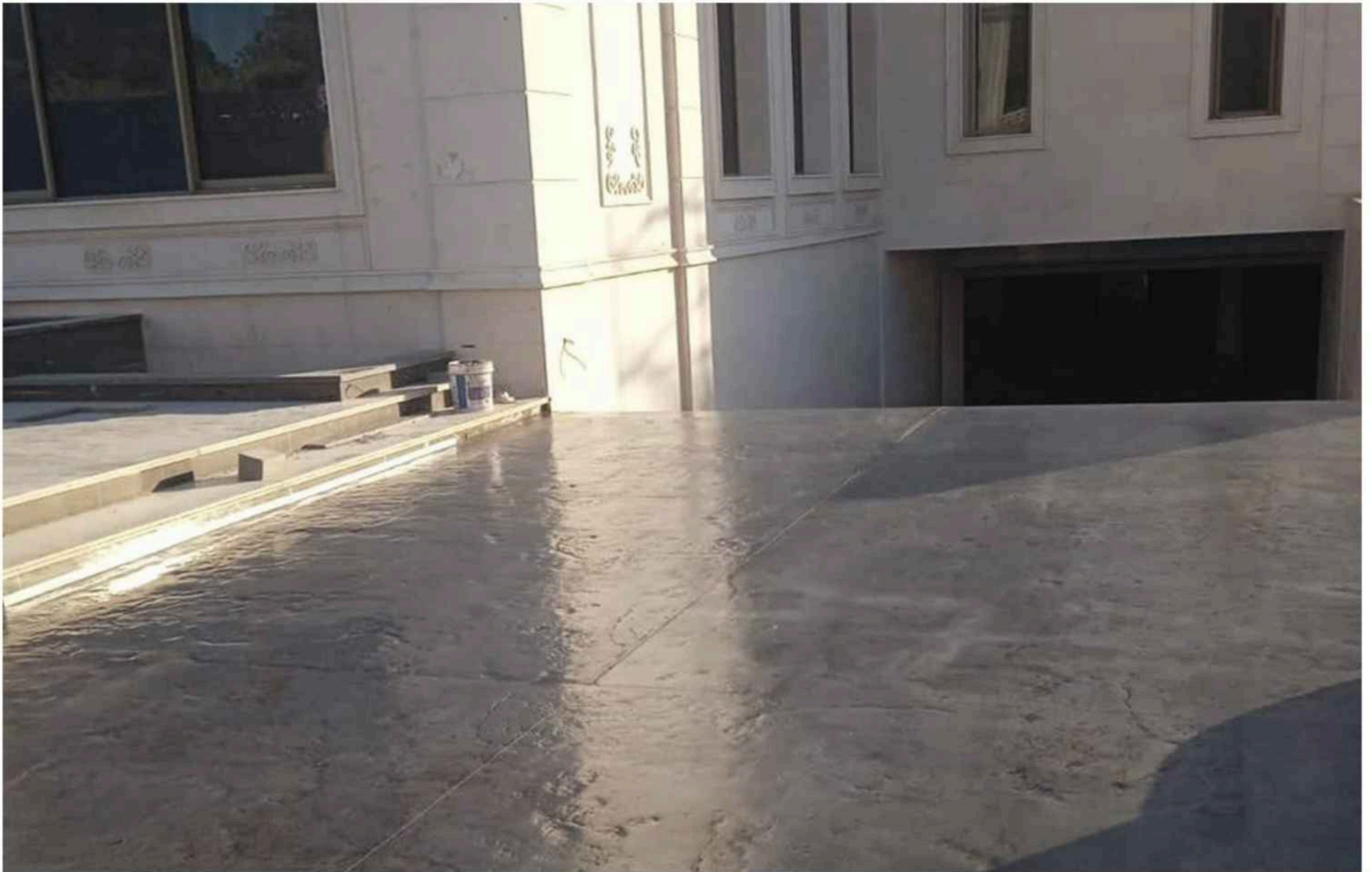
Stamped Concrete Work in Abu Dhabi
