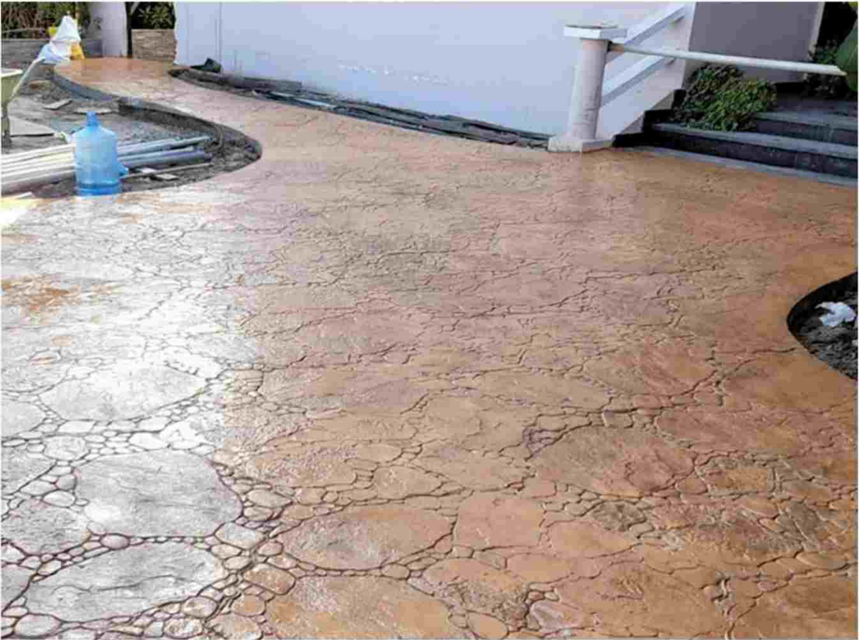
Stamped concrete work in The Villa, Dubai
