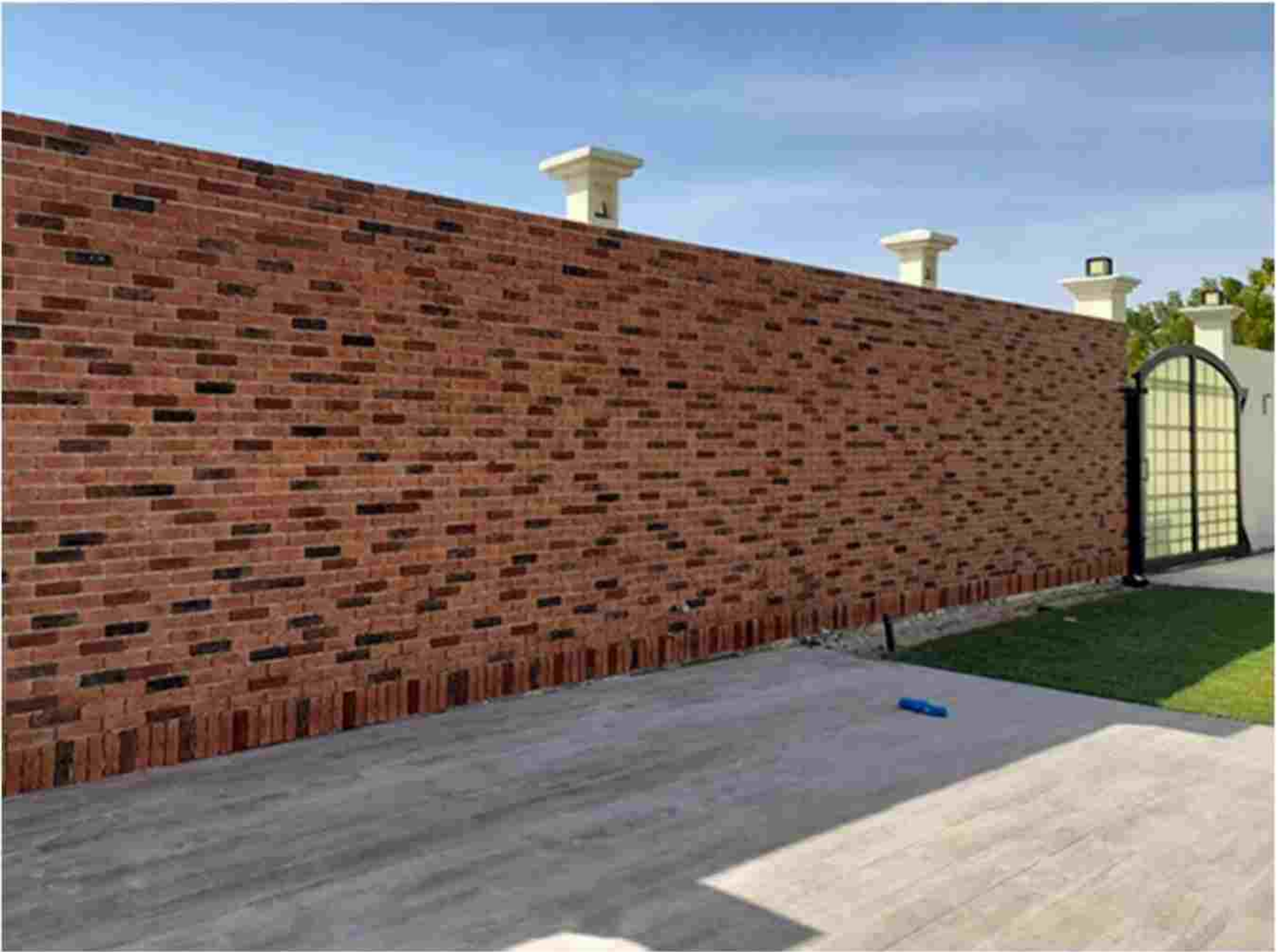
Brick work in Abu Dhabi
