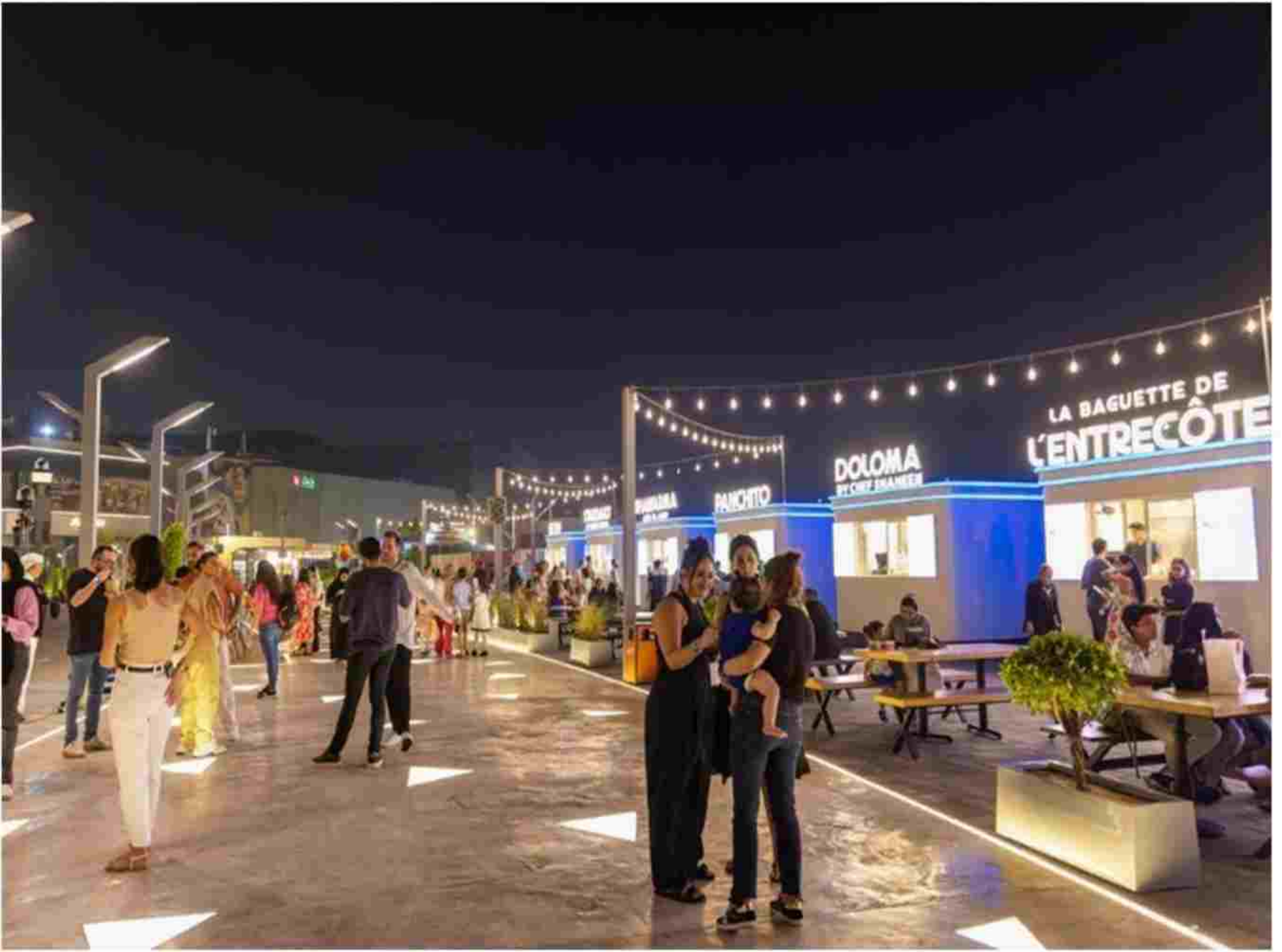
Stamped Concrete Work at The Bay By Social at Festival City
