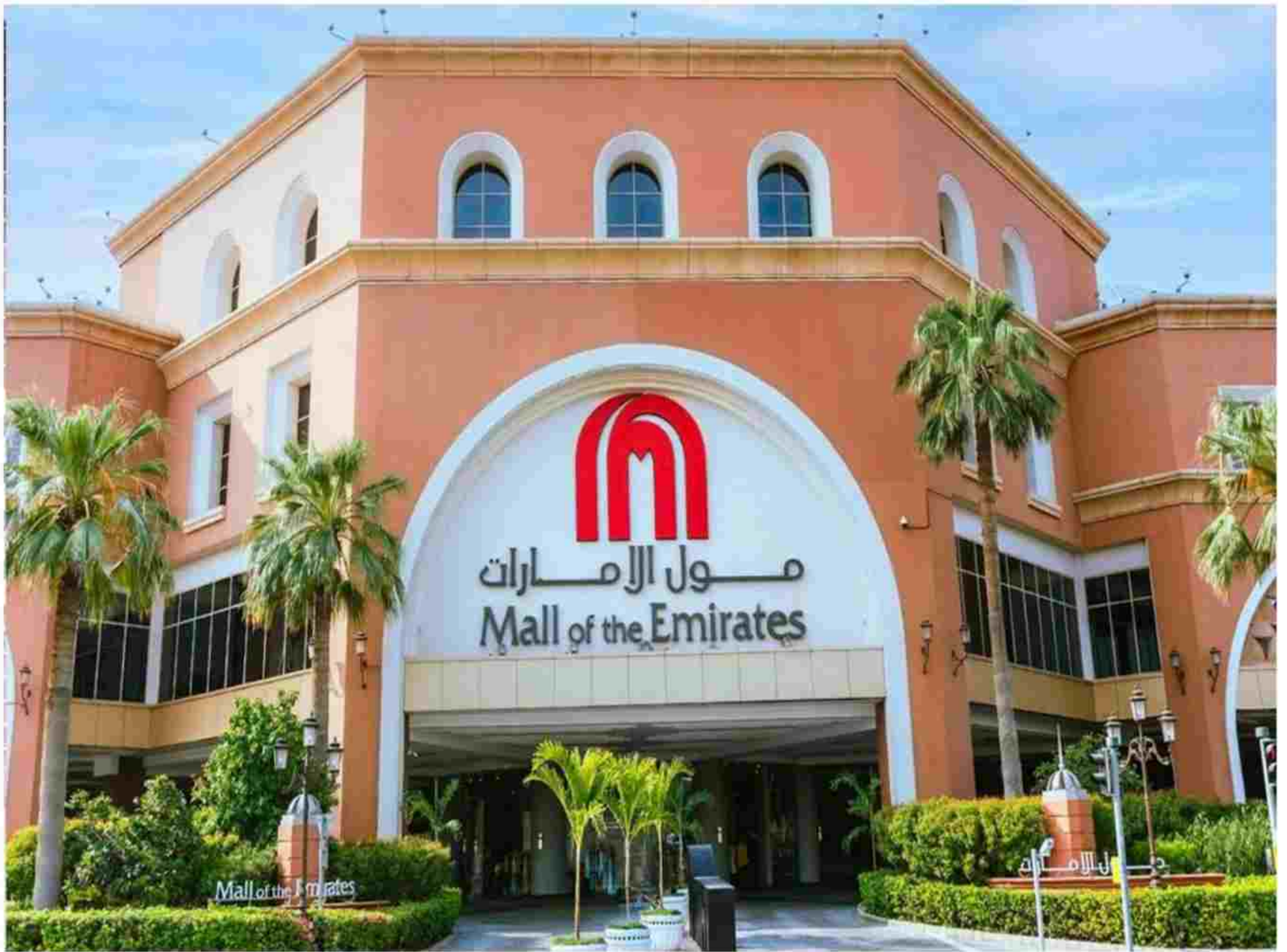
Brick Work Inside Mall of the Emirates
