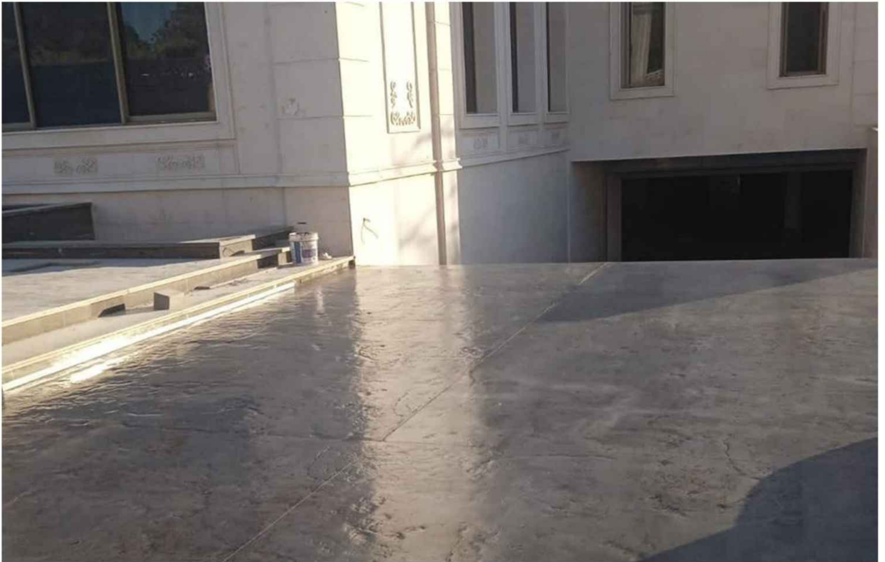
Stamped Concrete Work in Abu Dhabi
