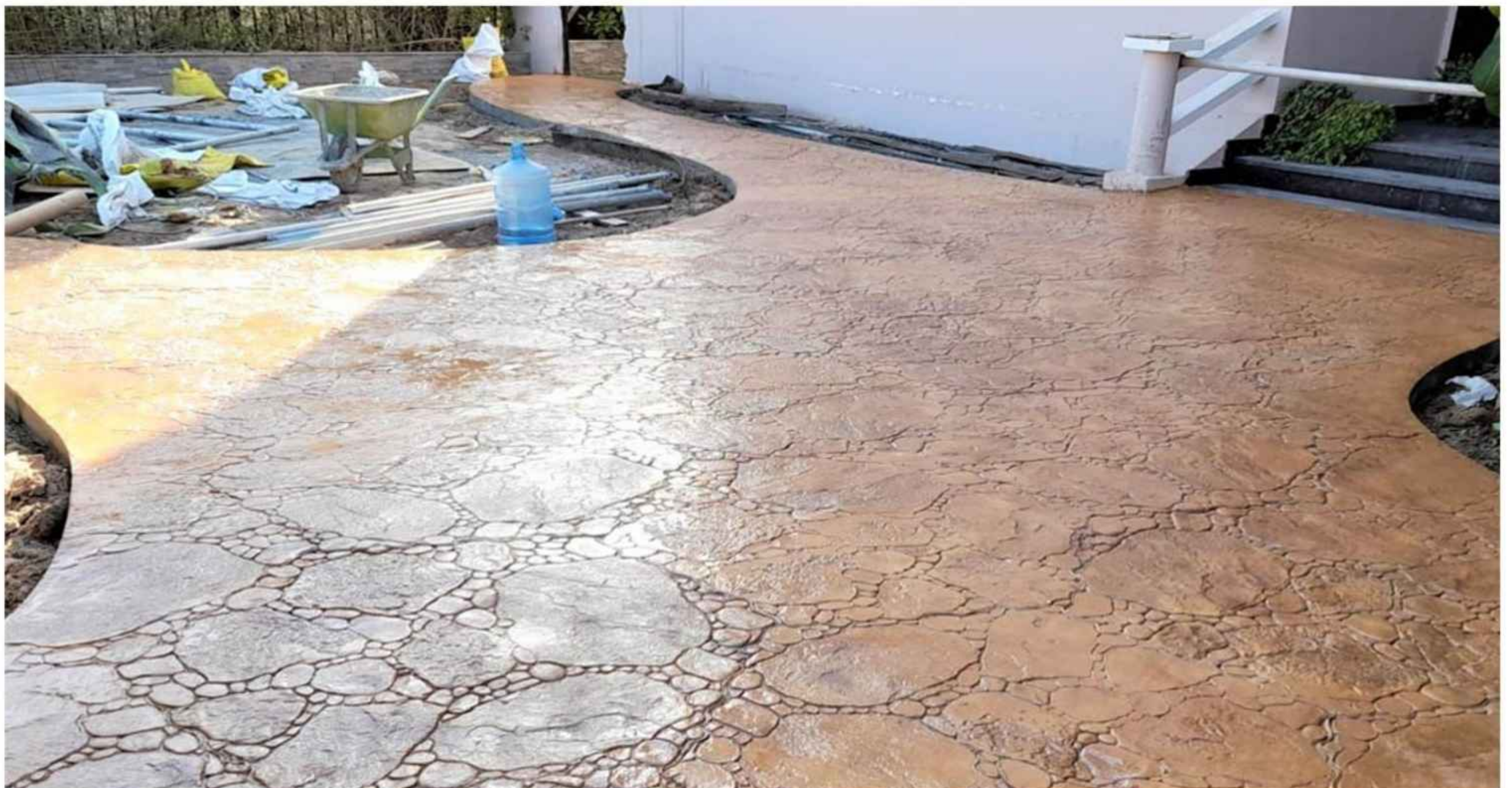
Stamped concrete work in The Villa, Dubai
