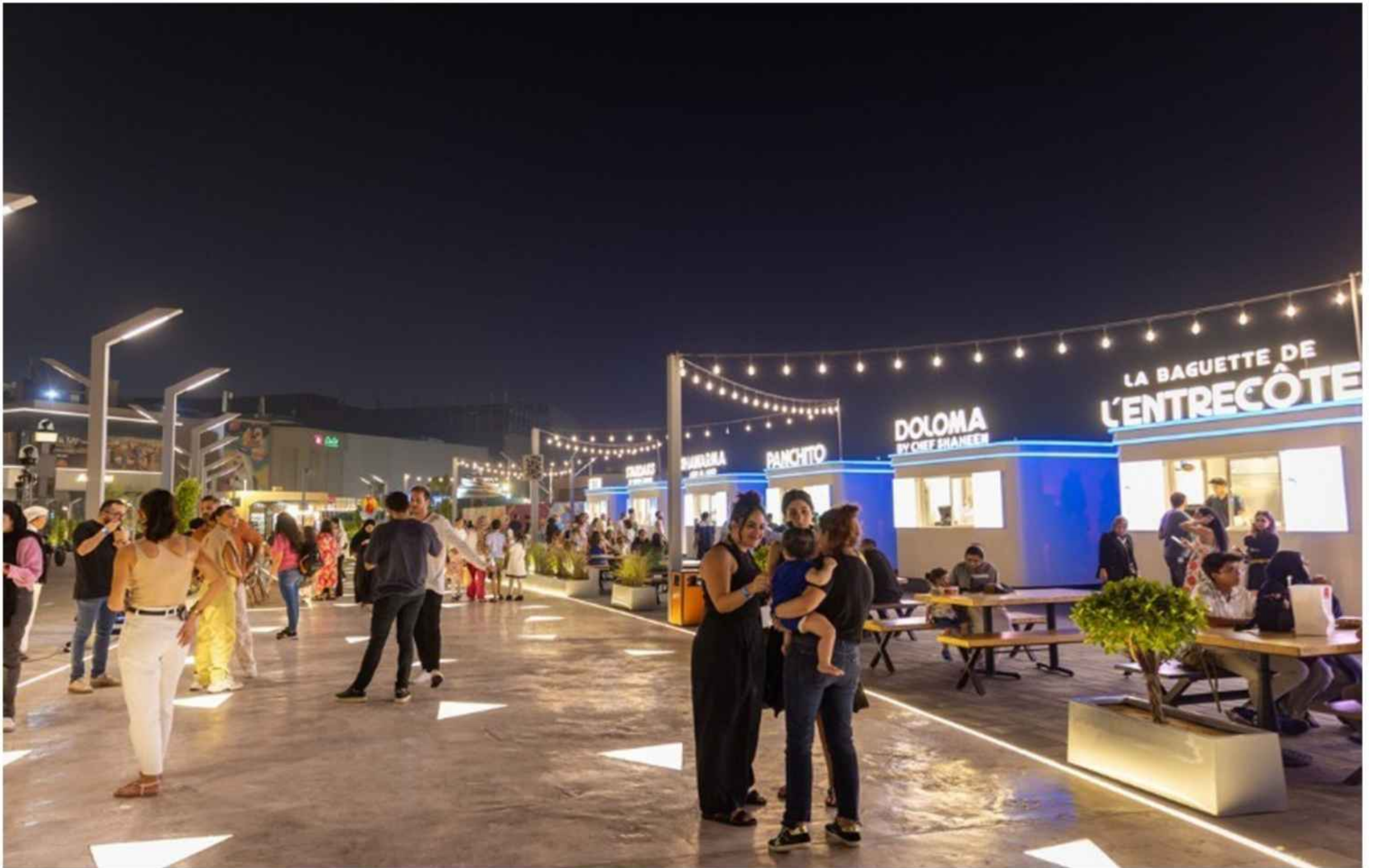
Stamped Concrete Work at The Bay By Social at Festival City
