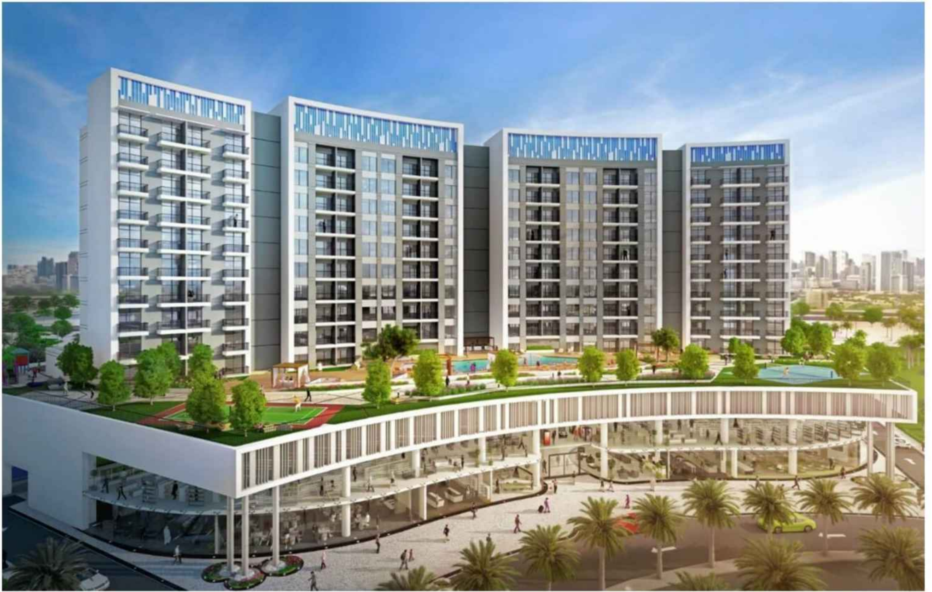
Stamped Concrete Work at Wavez by Danube
