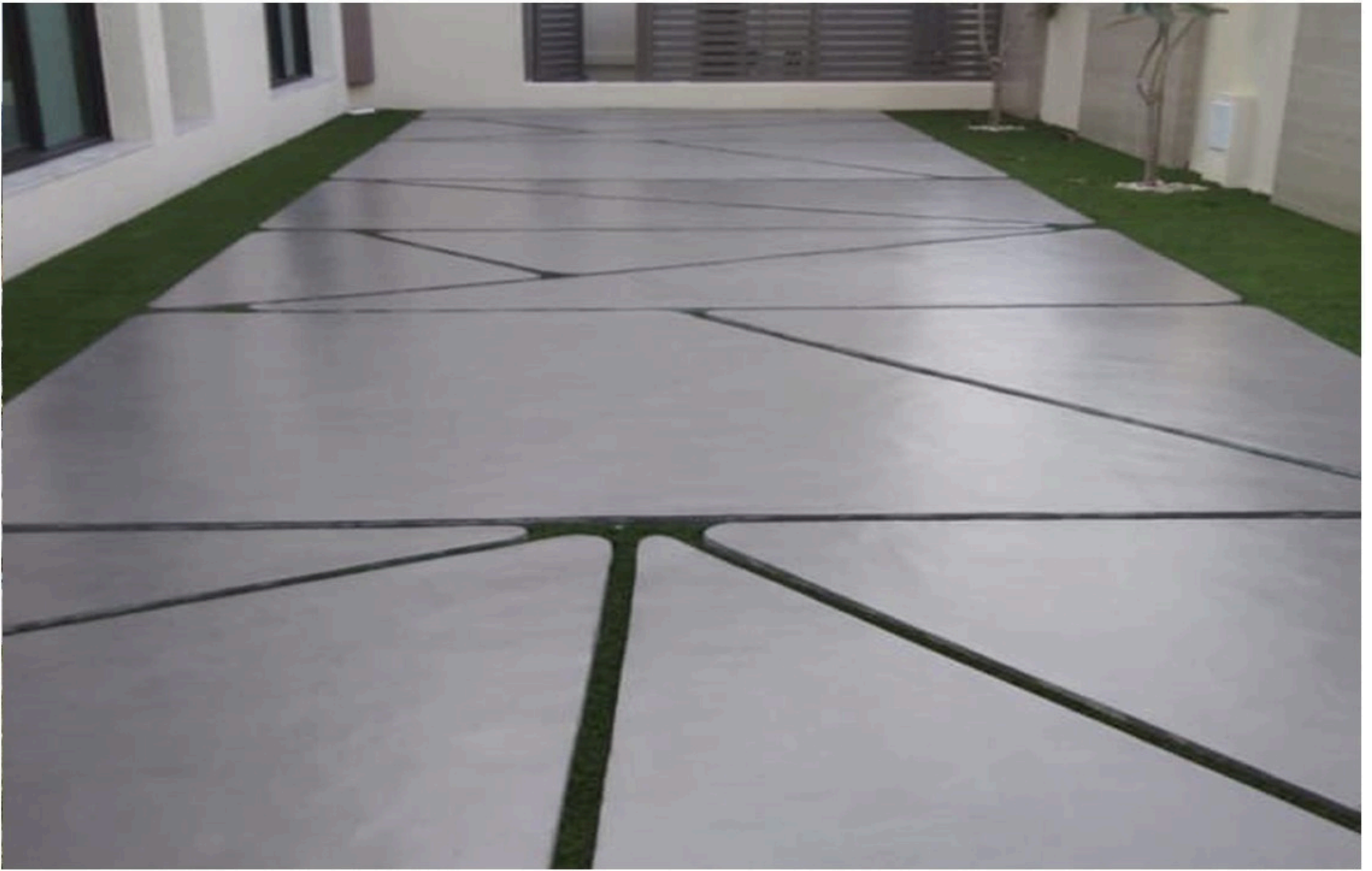
Microtopping Work at Dubai Sustainable City
