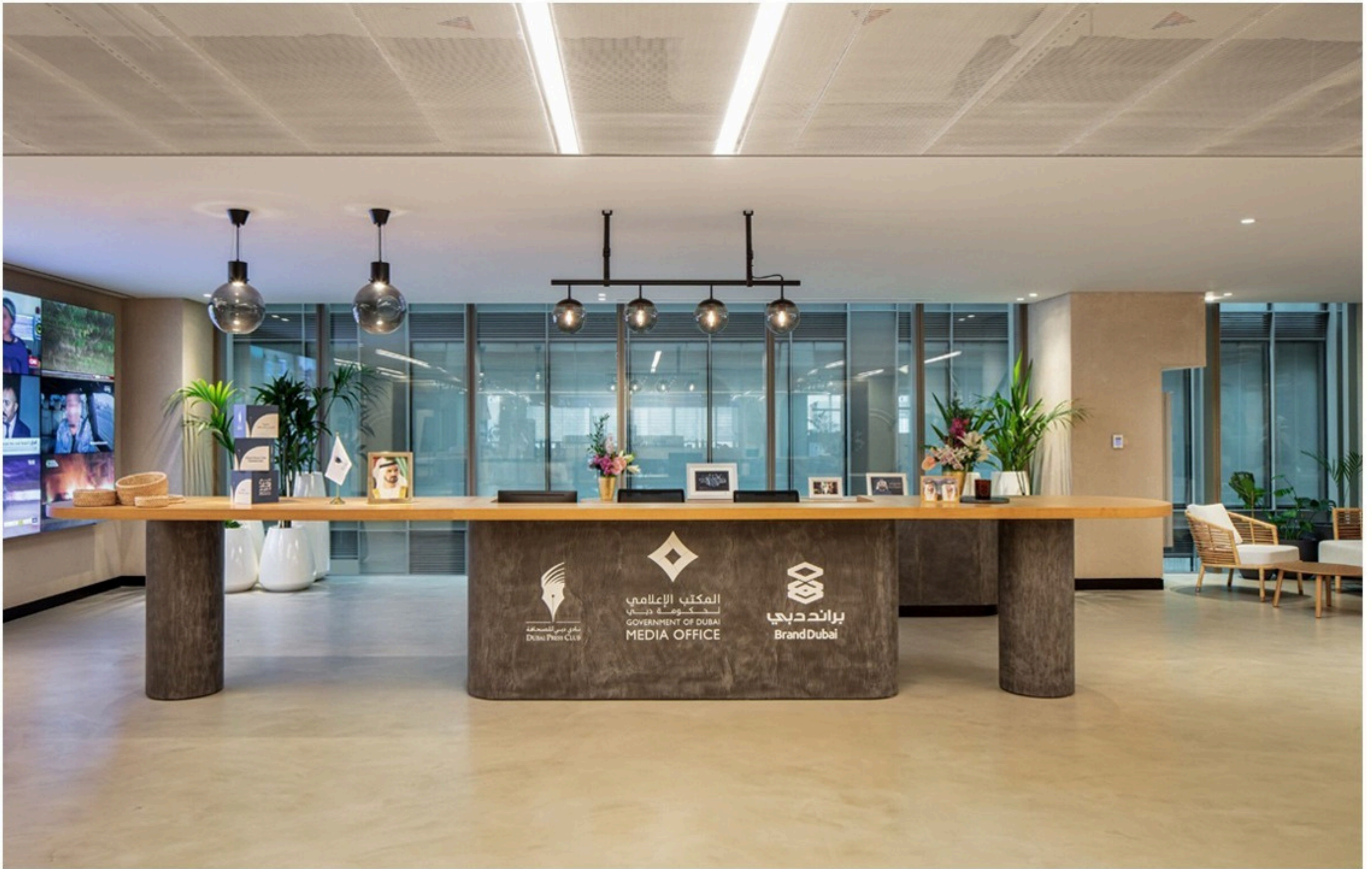
Microtopping Work at Government of Dubai Media Office
