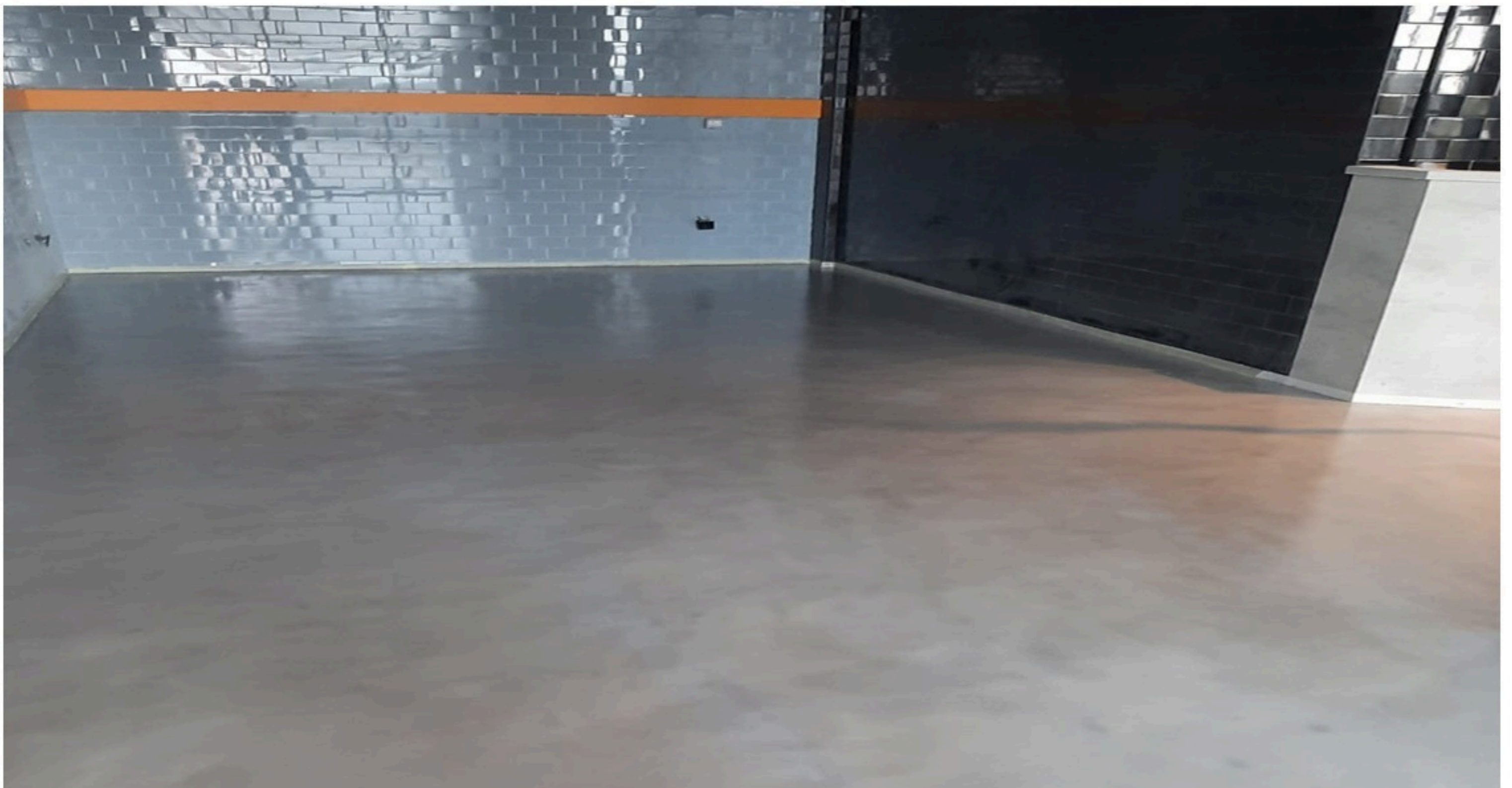
Microtopping Work at Coffee Shop In Khawanej
