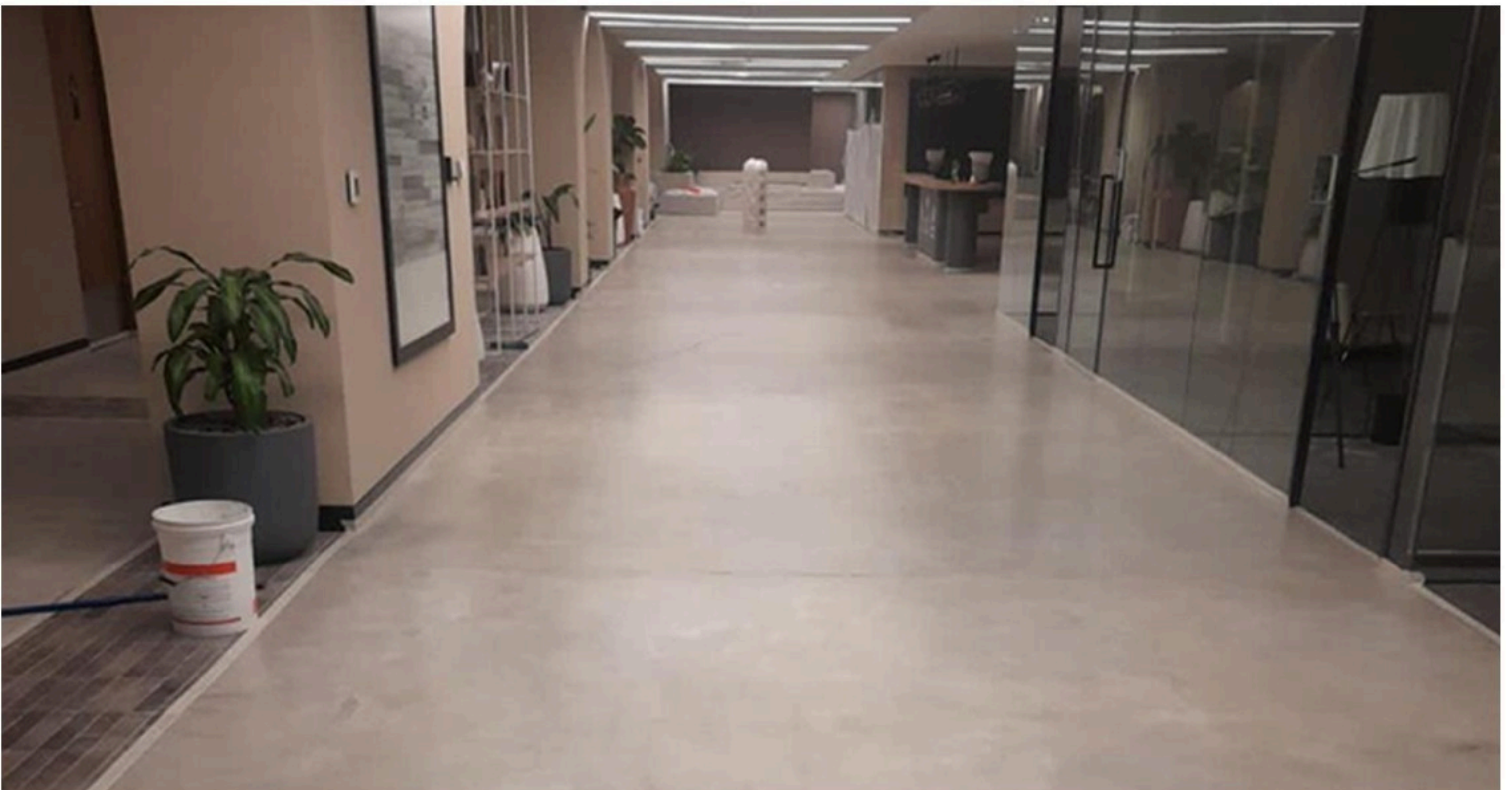
Microtopping Work in Dubai
