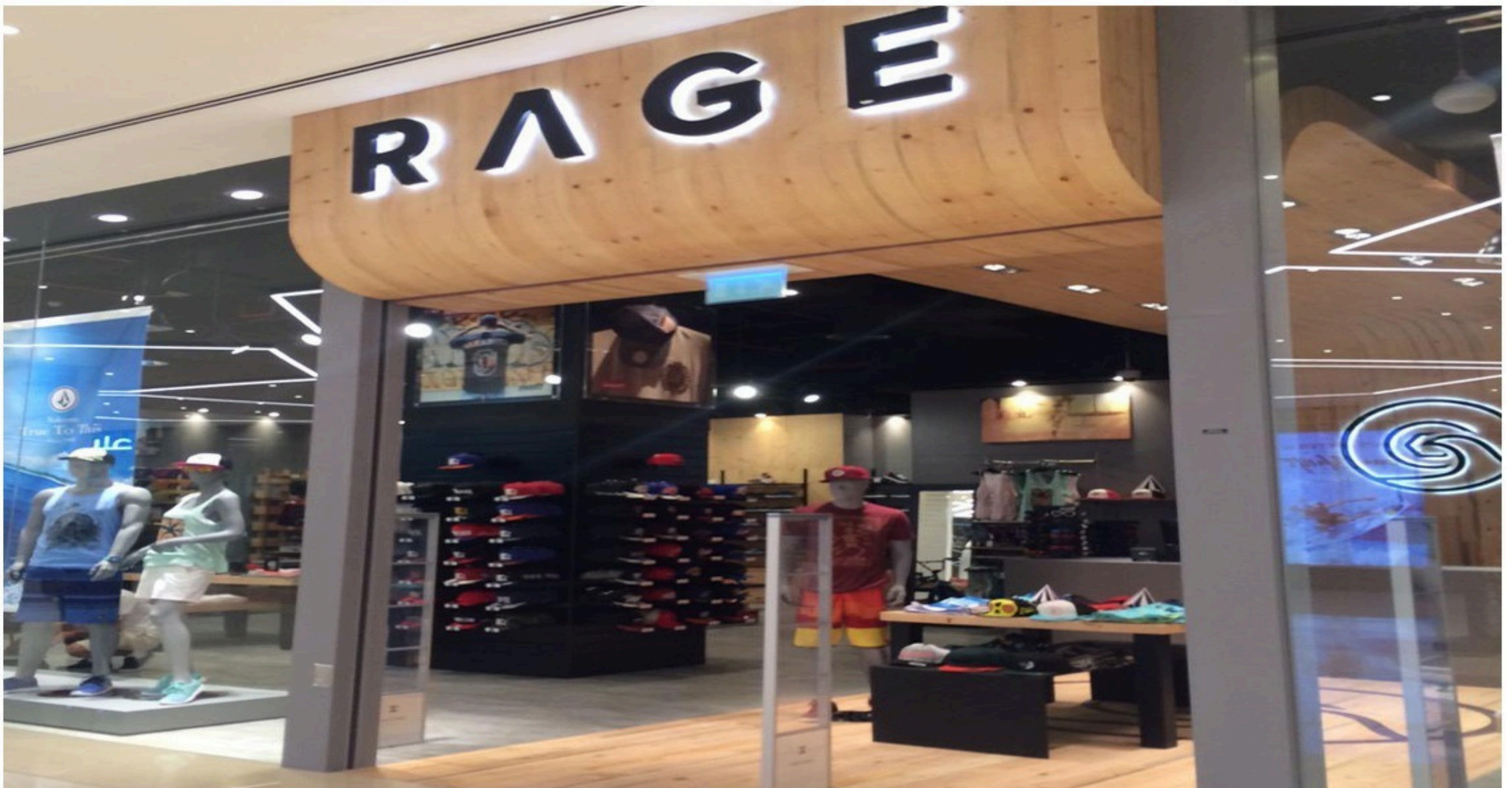
Microtopping Work at Rage Nakheel Mall
