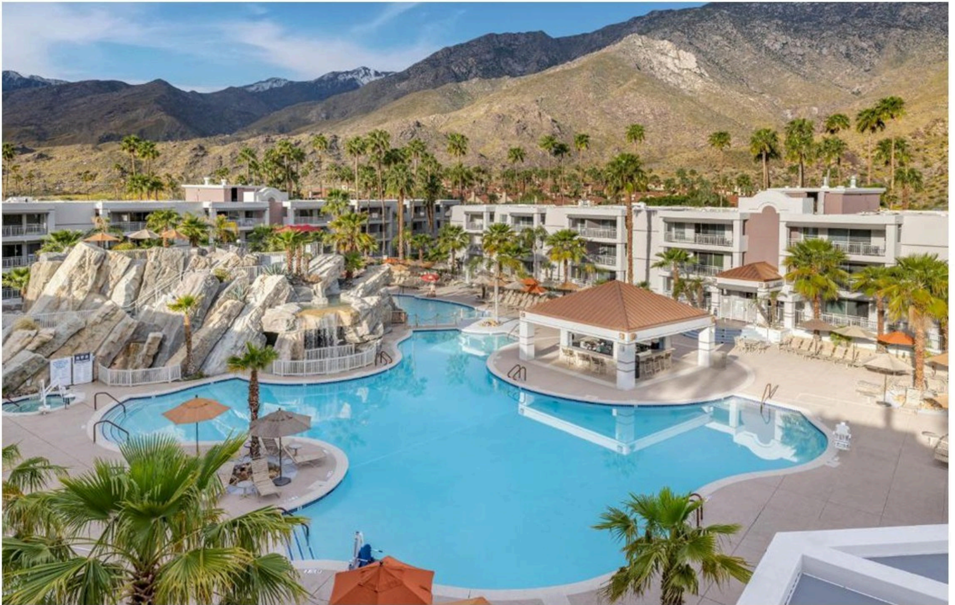
Microtopping Work at Canyon View Spa and Resort Oman for Arkan Majan International
