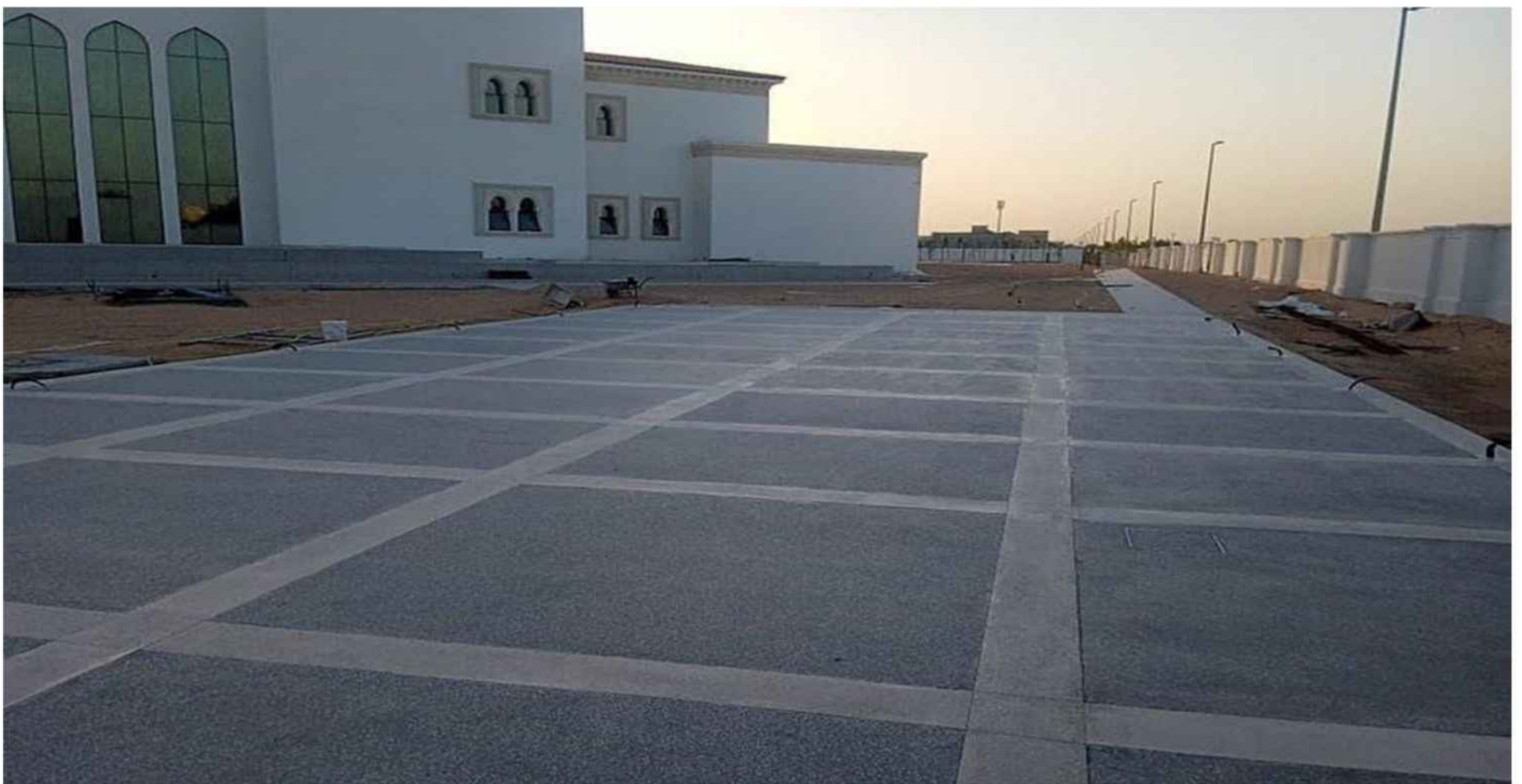
Exposed Aggregate Work at Sharjah Private Palace
