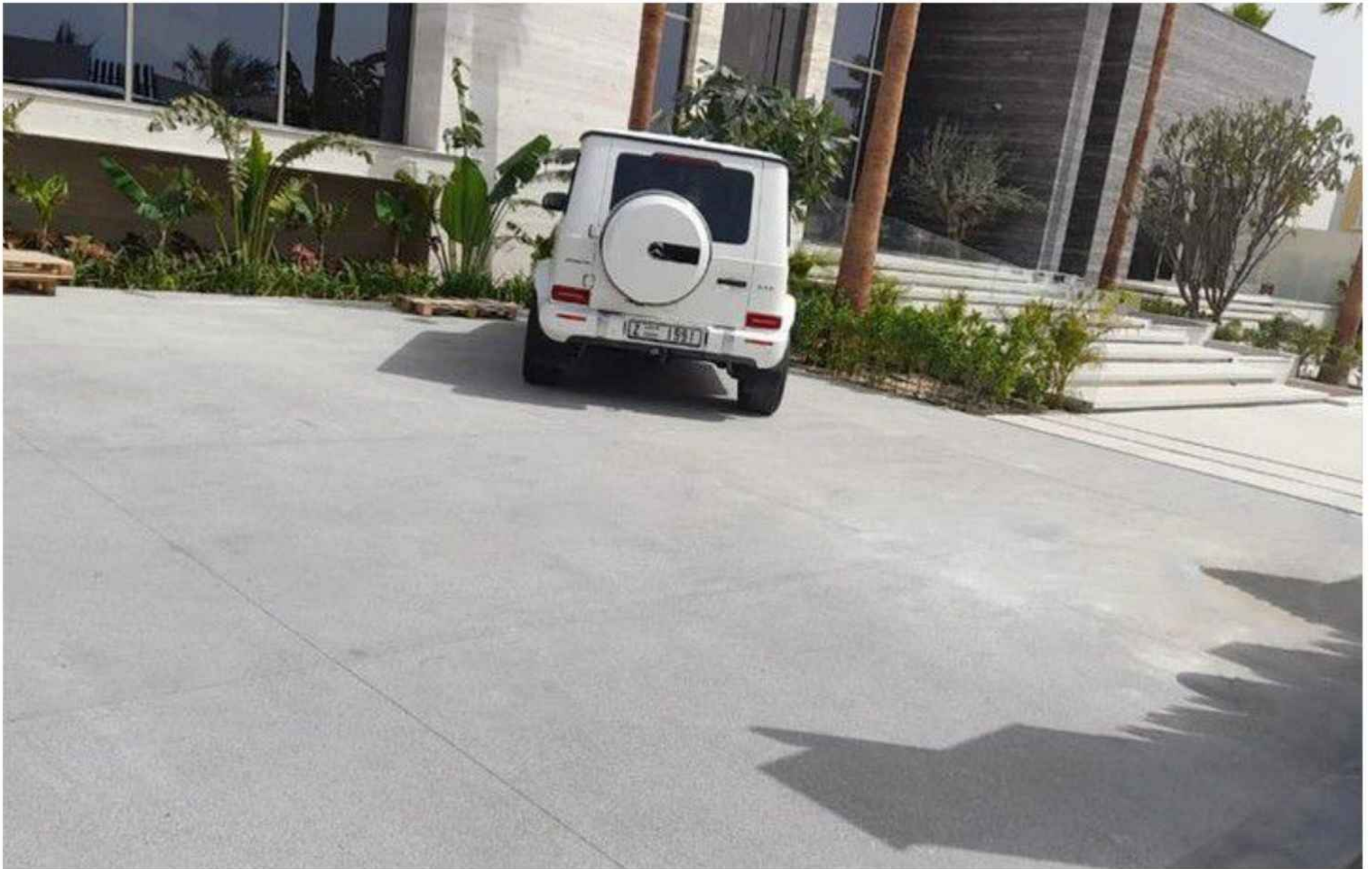
Exposed Aggregate Work at Nad Al Sheba Private Villa
