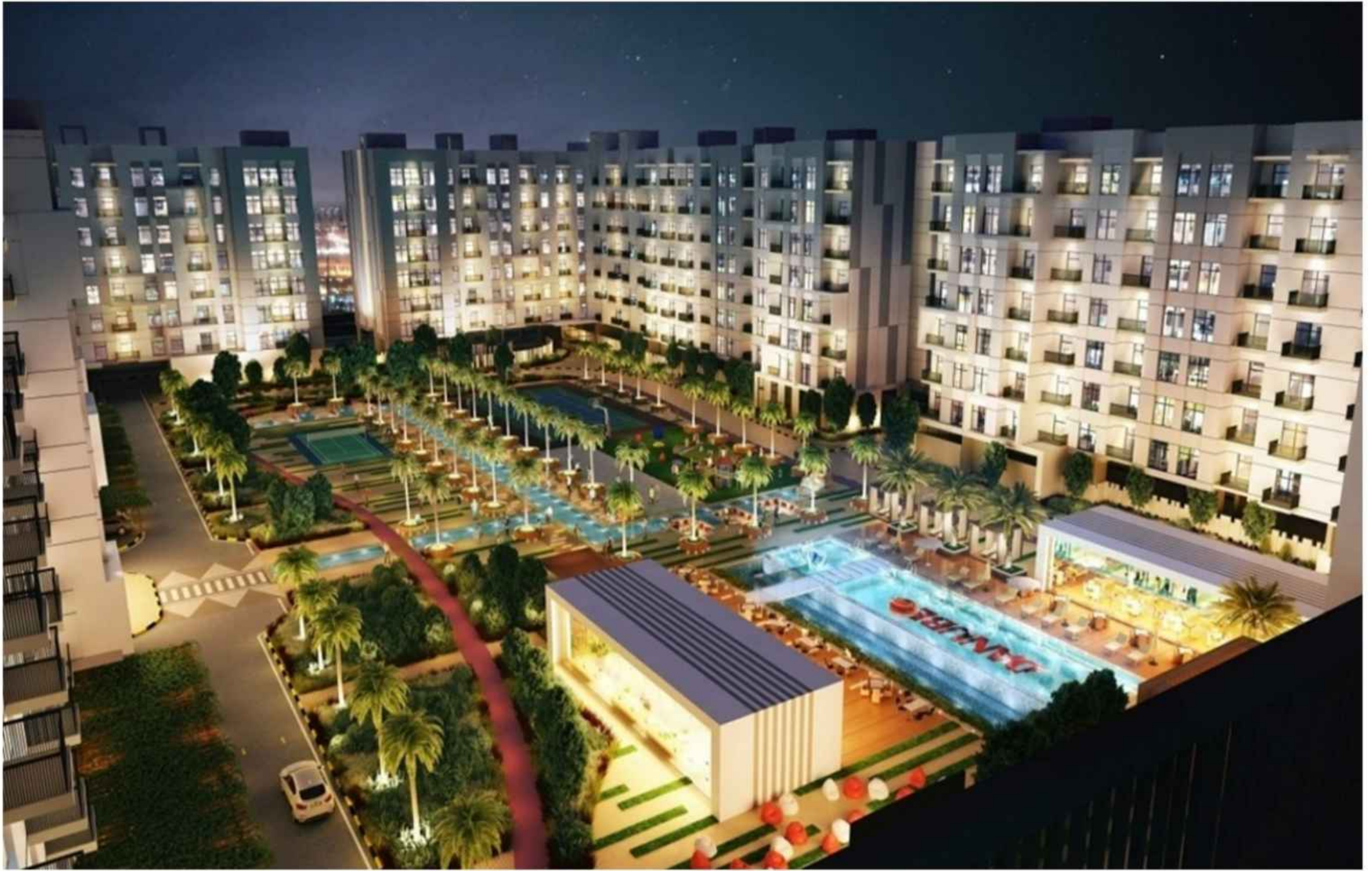
Exposed Aggregate Work at Lawnz by Danube
