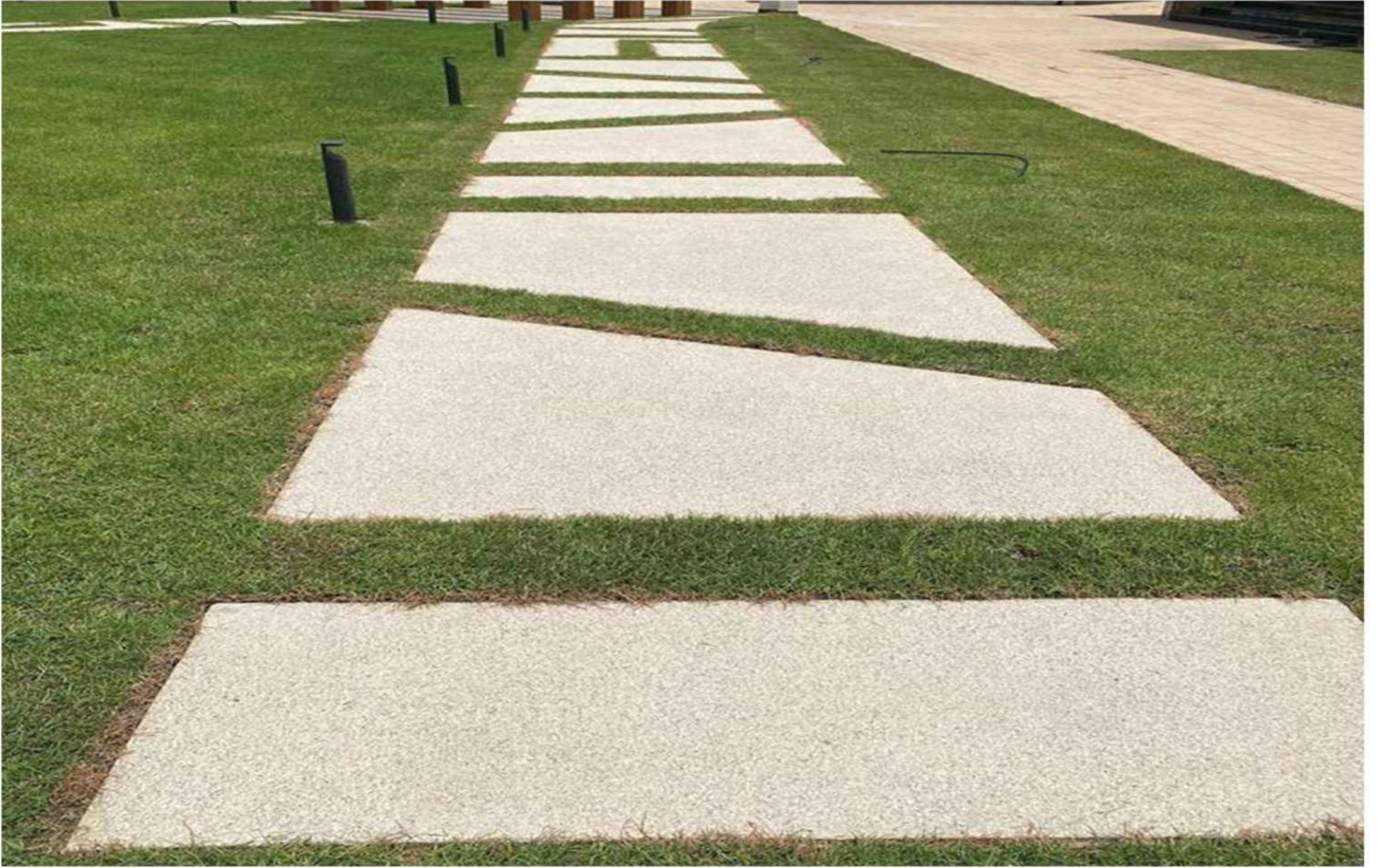
Exposed Aggregate Work at Nal Al Shiba
