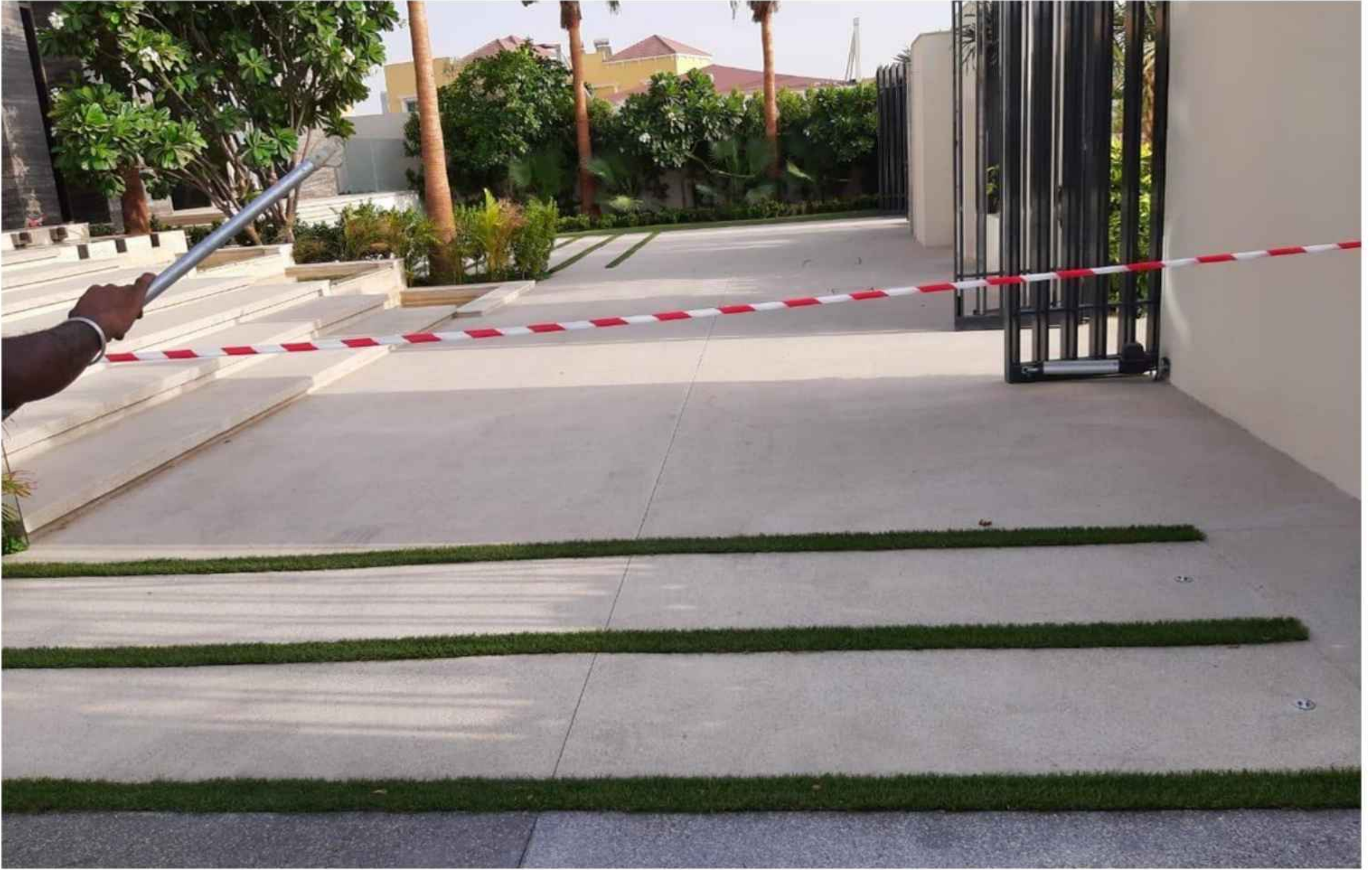
Exposed Aggregate Work at Nad Al Sheba
