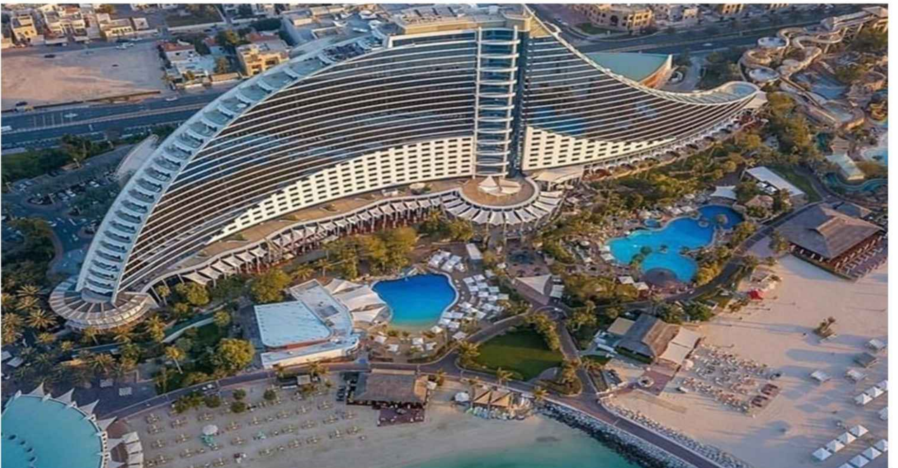
Exposed Aggregate Work at Jumeirah Beach Hotel
