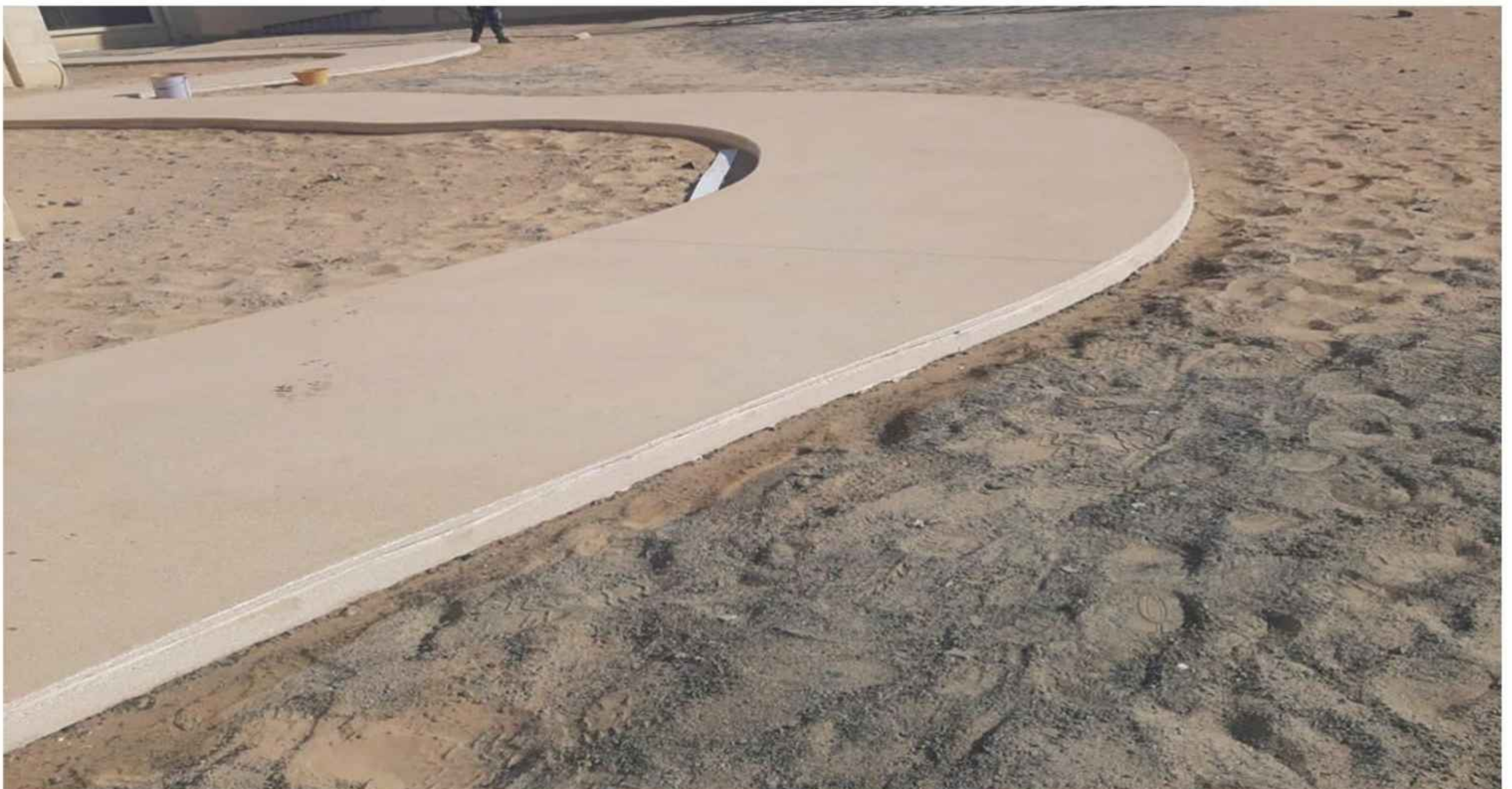
Exposed Aggregate Work at Private Villa
