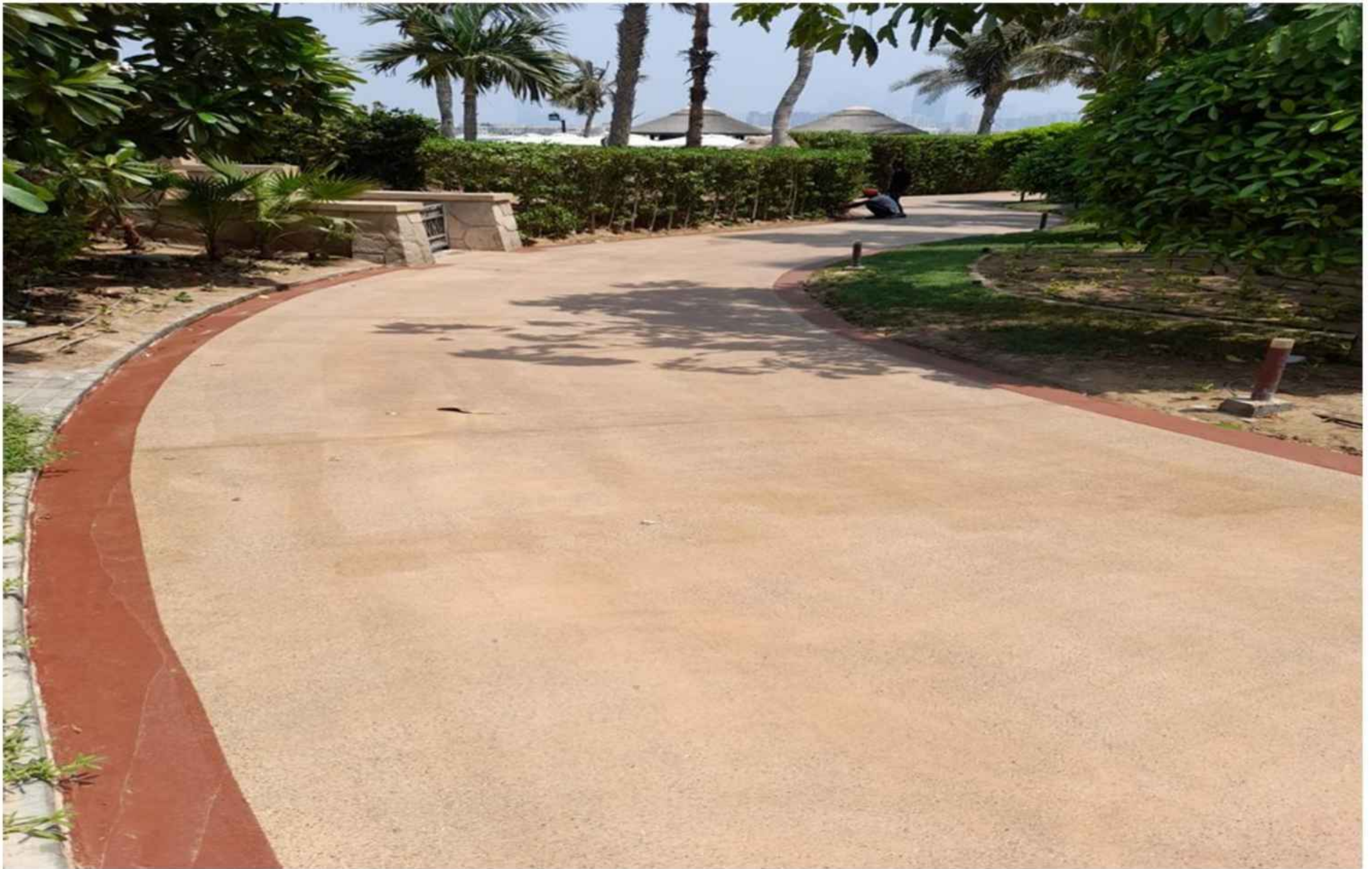
Exposed Aggregate Work at Sofitel The Palm
