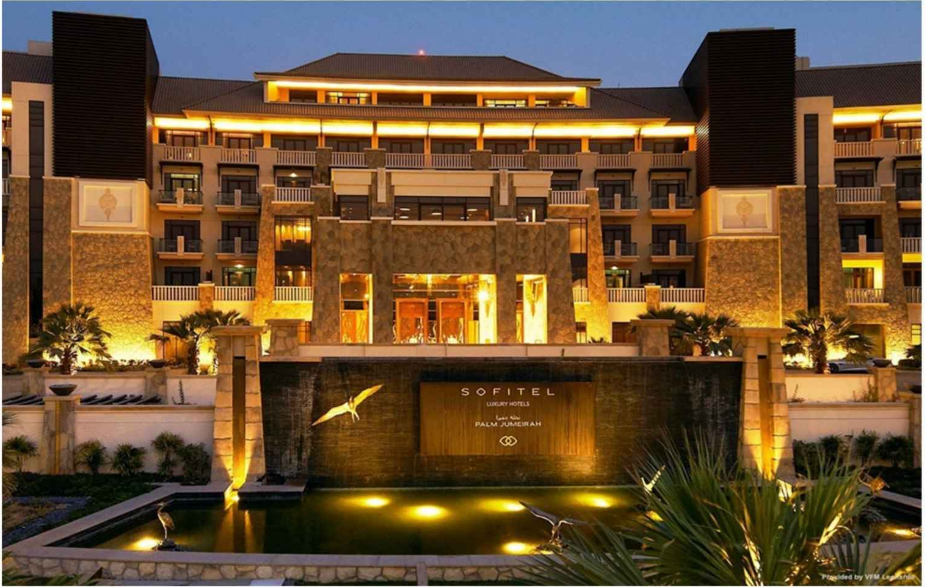
Exposed Aggregate Work at Sofitel The Palm
