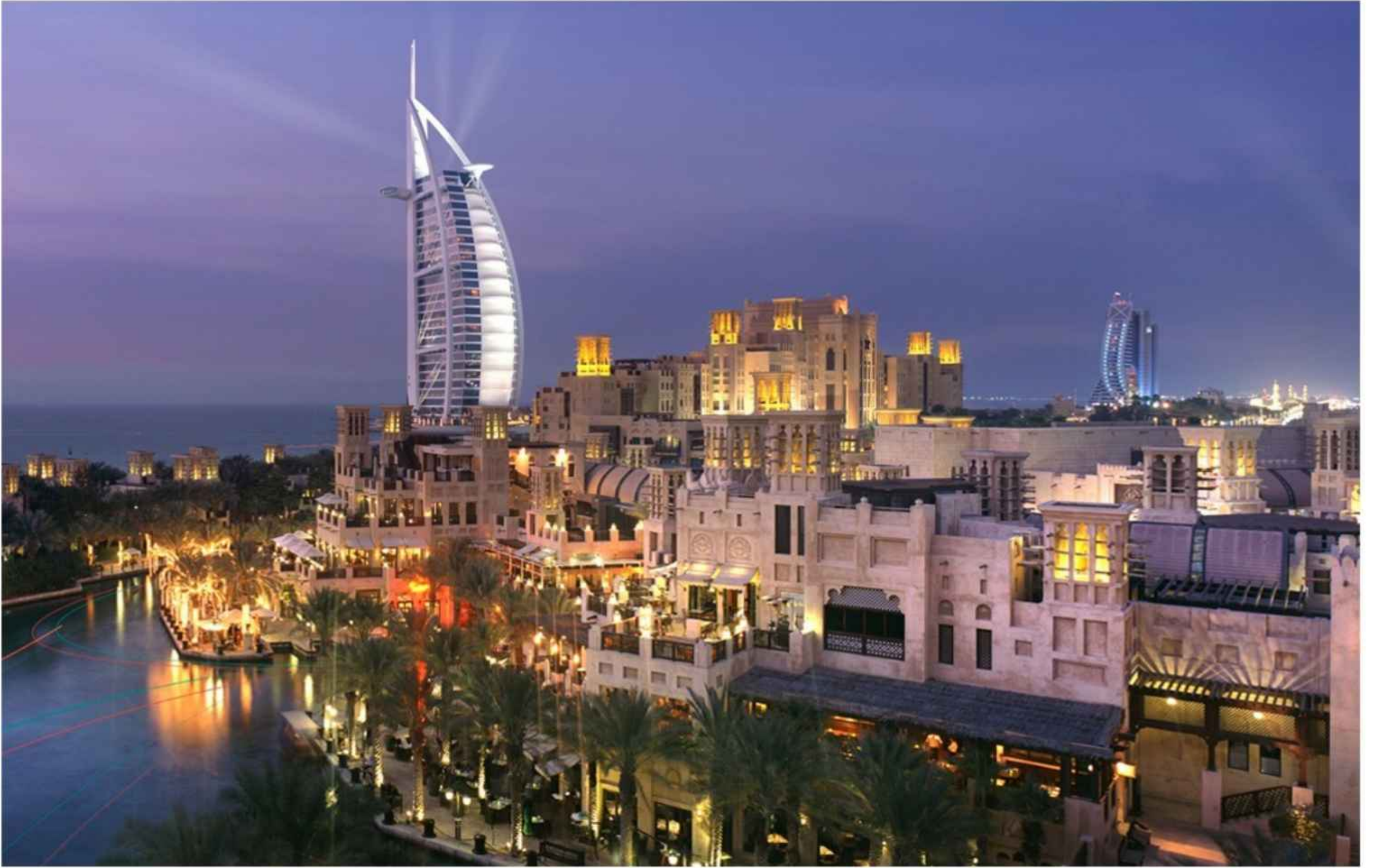
Exposed Aggregate Work at Souq Madinat Jumeirah
